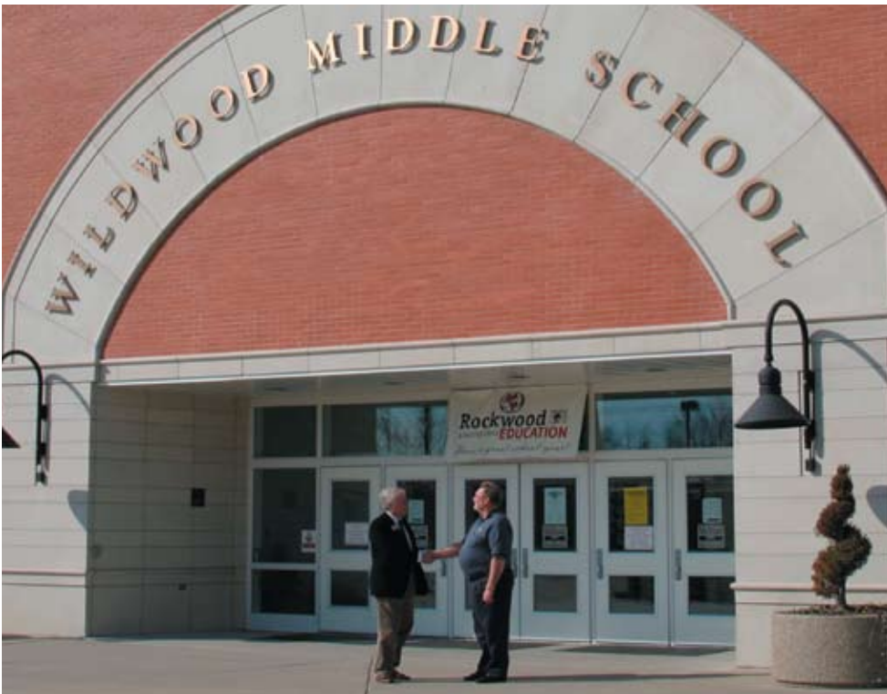
Rockwood School District depends on H 2 Orange 2 117 to assure a clean and sanitized environment for all its students, including those with compromised immune systems and special medical needs.
